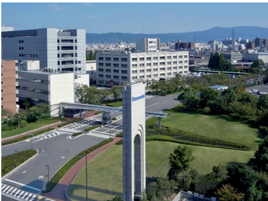
Panasonic, Electric Works Company (Osaka, Japan)
