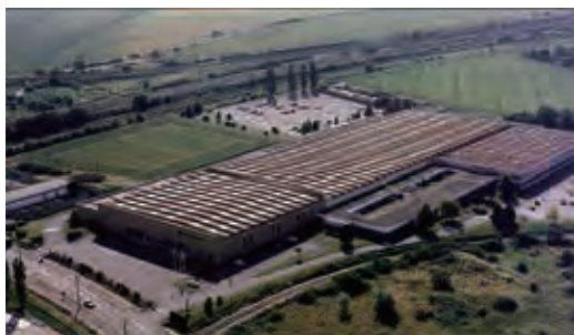
Canlis Factory, Dijon, France
