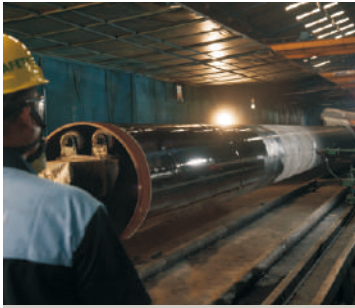
External Epoxy Coating
